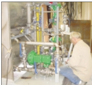
The Process Trainer for ExxonMobil's Zafiro FPSO under construction at BTTC.
